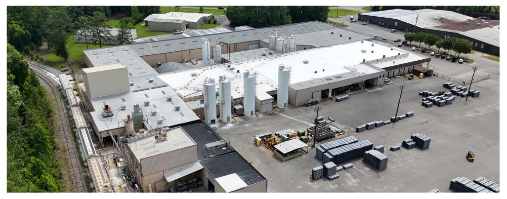
For this commercial roofing project at Atkore International in Thomasville, GA, we installed a 190-square roofing system designed for durability and energy efficiency. The project included the installation of 2" Polyiso insulation, providing excellent thermal resistance and reducing energy costs for the facility.
