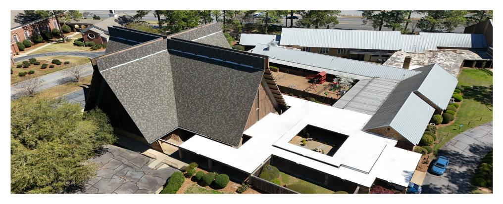
This project at Covenant Presbyterian Church in Albany, GA involved a full roof replacement following wind damage sustained during a storm in 2019. We removed the existing roofing system and installed approximately 600 squares of architectural shingles to restore the building's integrity.
