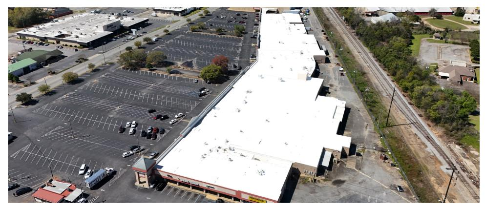
This project at Brooks Plaza in Albany, GA involved a complete re-roof of the commercial retail center. We installed 2,320 squares of .60 mil TPO roofing membrane, replacing the existing system with a more modern, energy-efficient solution.
