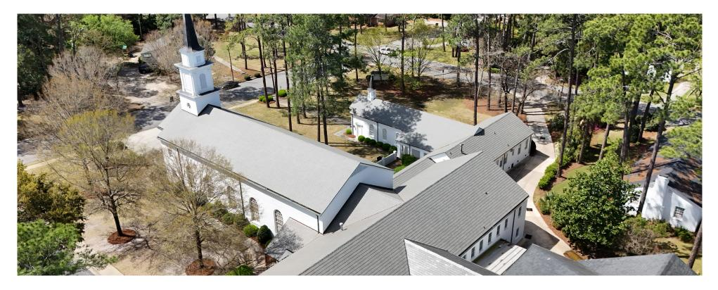
This project at Trinity Baptist Church in Moultrie, GA involved a complete replacement of the existing slateroofing system. Our team removed the old roof and installed a new composite slate roofing system, bringing the building up to current standards with improved protection and appearance.
