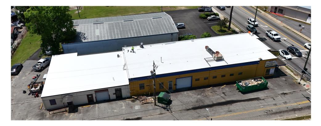
This project at Beds for Less in Valdosta, GA consisted of a full commercial roof replacement. Our team removed the aging torched-down roofing system and installed approximately 85 squares of GAF 60 mil TPO membrane to modernize and protect the building.
