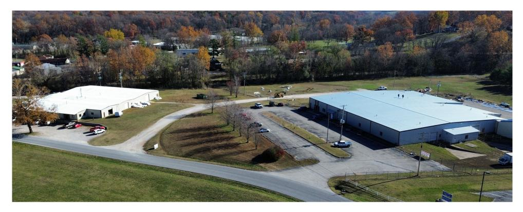
This project at Iron Mule in Cassville, MO involved a full replacement of the metal roofing system after the building sustained significant hail damage. We removed the damaged roof and installed approximately 1,200 squares of 26-gauge R-panel metal, restoring full protection to the facility.
