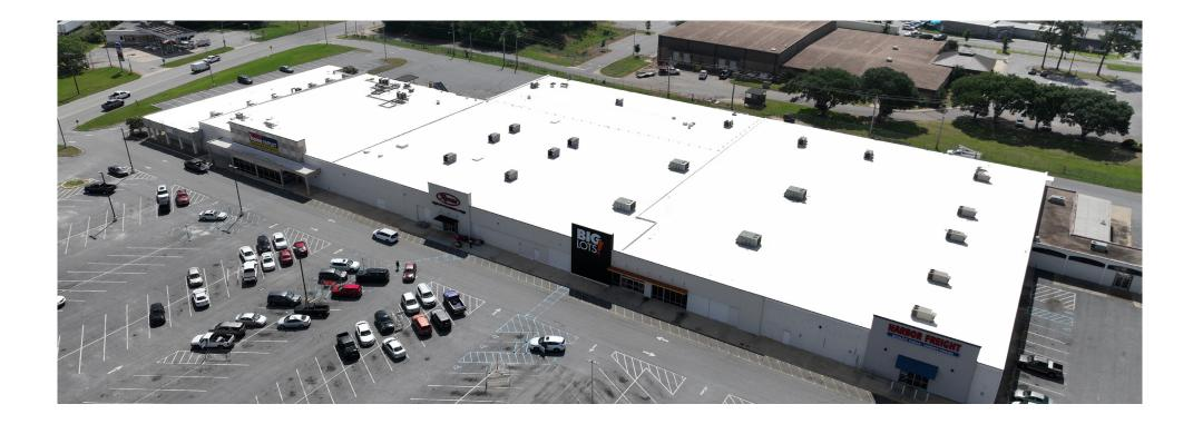
This project at Harbor Freight in Albany, GA involved a complete roof replacement of the retail facility. We removed the existing roofing system and installed approximately 540 squares of GAF 60 mil TPO membrane.
