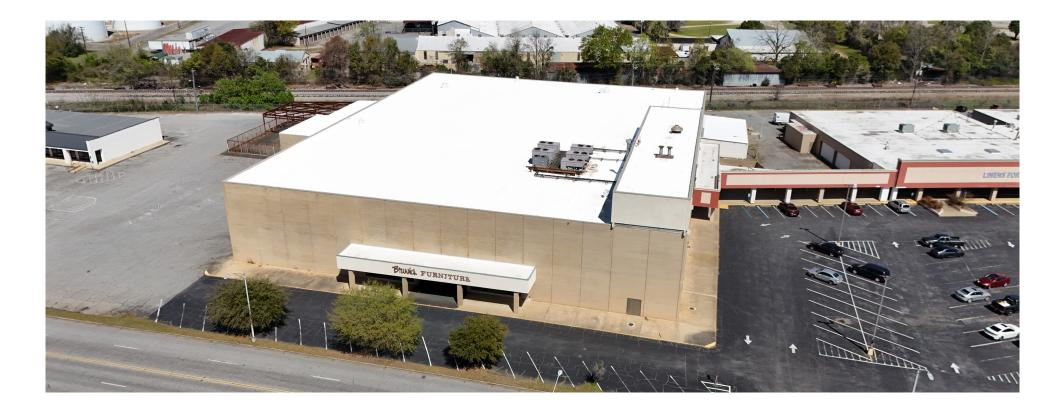
At Brooks Furniture in Albany, GA, we completed a full roof replacement, covering 612 squares with a new 60 mil TPO roofing system. The existing roof was removed and replaced with a fully adhered TPO membrane, chosen for its excellent durability, energy efficiency, and low-maintenance performance.
