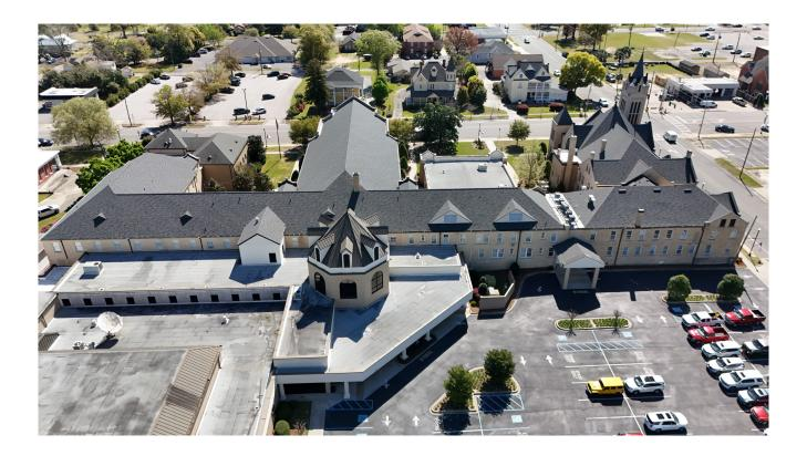
This project at First Baptist Church in Tifton, GA involved a complete re-roof of the main church building. We removed the existing roofing system and installed 450 squares of architectural shingles, restoring the roof with a durable and updated replacement.
