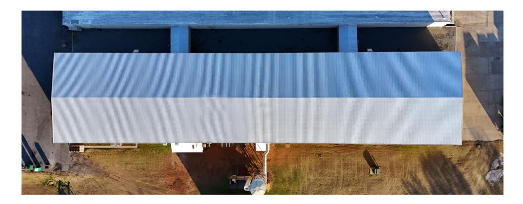
This project at Synergy Peanut in Tifton, GA involved a full replacement of the facility's metal roofing system following hail damage. We removed the existing panels and installed approximately 340 squares of new 26-gauge metal roofing.
