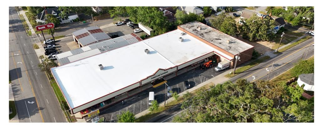
This project at Furniture Express in Valdosta, GA involved the removal of the existing torched-down roofing system and installation of a new single-ply membrane. We replaced the roof with approximately 243 squares of GAF 60 mil TPO, providing a modern, energy-efficient solution.
